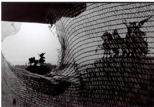
Godess of Nike, repair works on the rooftop, Parliament, Vienna, Austria, 2004 © Christine de Grancy / AnzenbergerGallery
